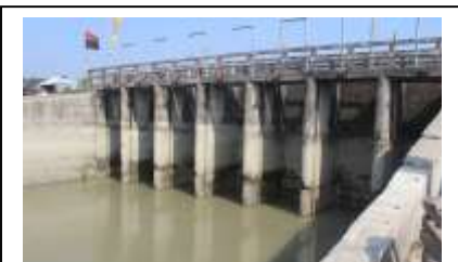
Gabtohi sluice (7-vents) built by CDSP III in 2009 still operational, but at risk of erosion
