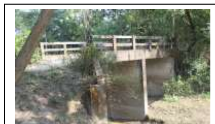
A culvert built by CDSP located at Mir somaj, 1 no. Horni Union Parishod, Boyer
